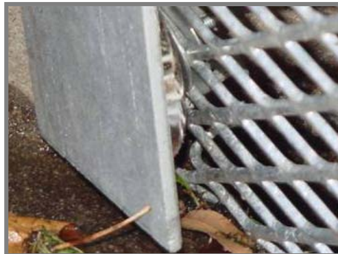
Figure 1.5 Typical Opening Screen Cover Magnet Locking Mechanism
