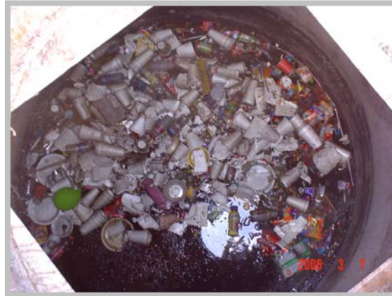
Figure 3.4 Typical CDS unit contents after storm event
