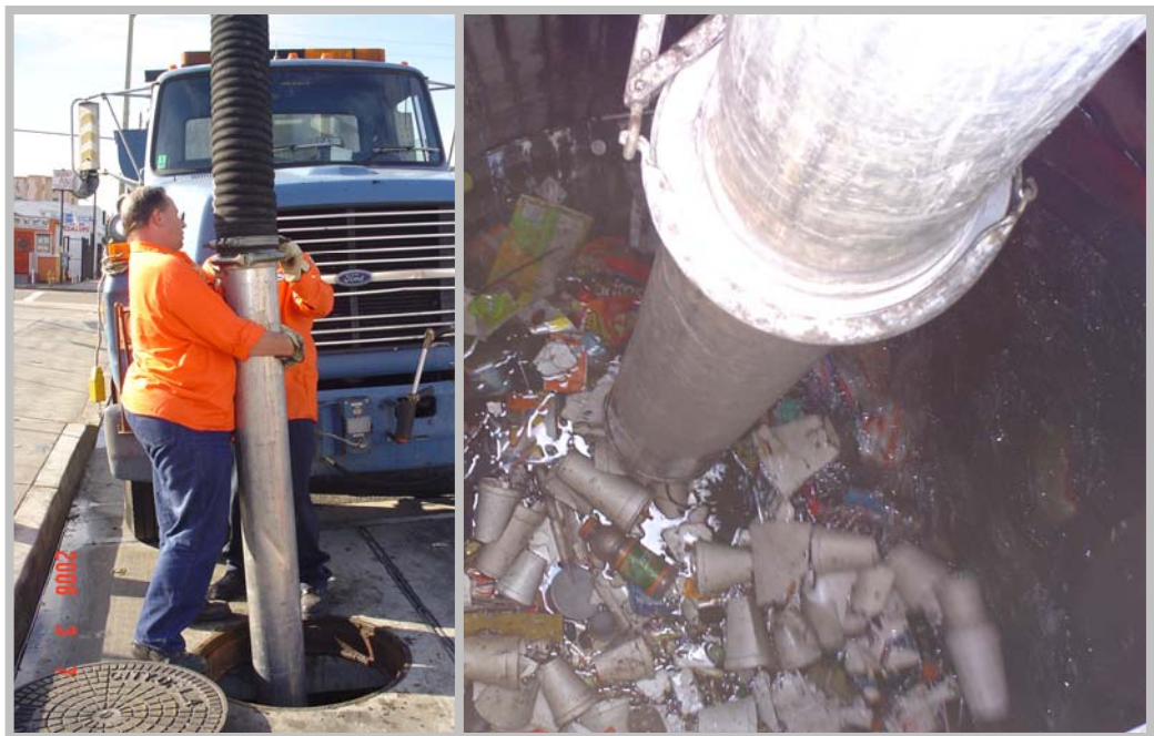
Figure 3.5 WCS D crews cleaning the CDS unit after a storm event
