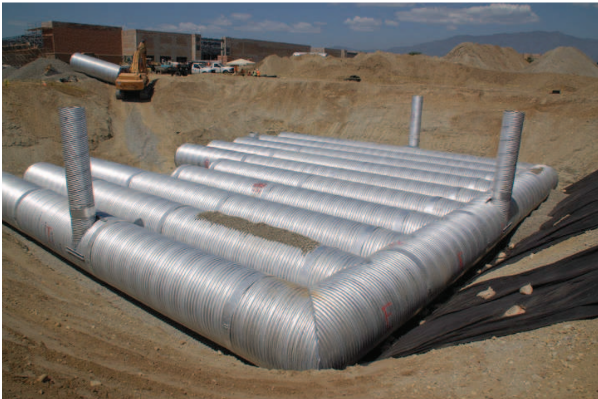
Figure 4-9 Photograph Storage/Detention System Using CMP (Contech, 2015)
