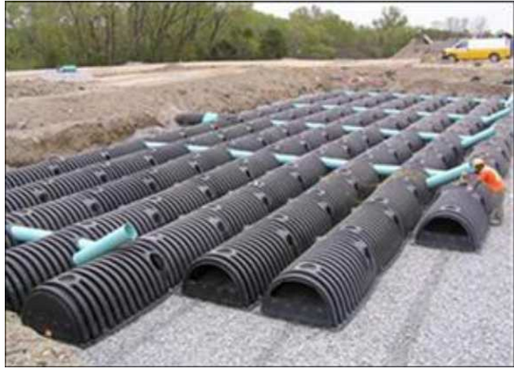
Figure 5-5: Example of StormChamber Units
