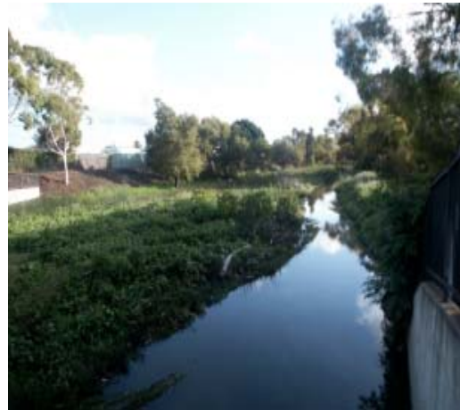
Wilmington Drain looking downstream from Lomita Boulevard
