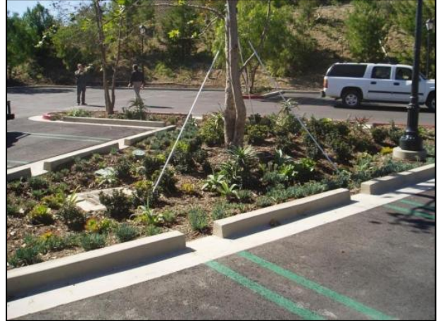
Bioretention in a Parking Lot
