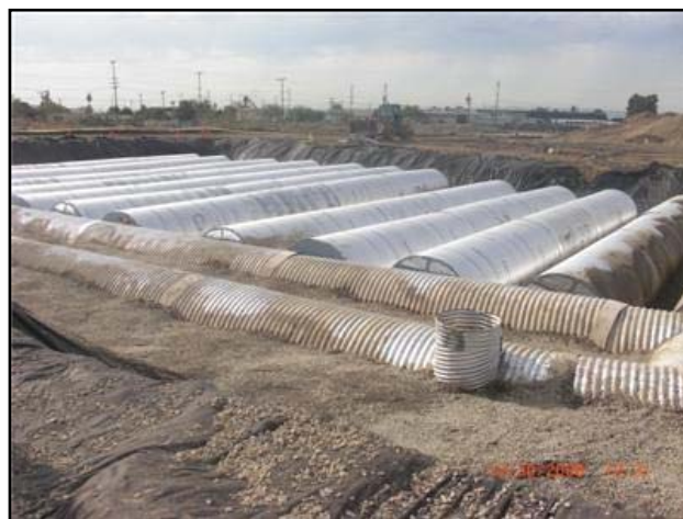
Underground Infiltration Units Lowe's, Pacoima
