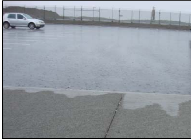
Permeable Pavement Application
