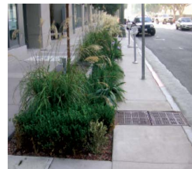
Parkway Infiltration Swale at 11 th St & Hope St - Los Angeles
