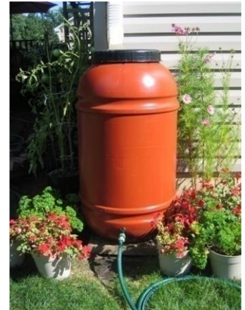
Downspout connection to Rain Barrel - Mar Vista Area
