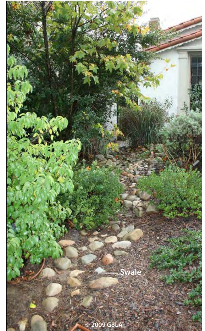
A swale directs water from the downspout to the rain garden. Many swales use rocks that create a dry creek bed look.
