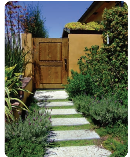
Grass Paver Block Walkway Photo Credit: City of Los Angeles
